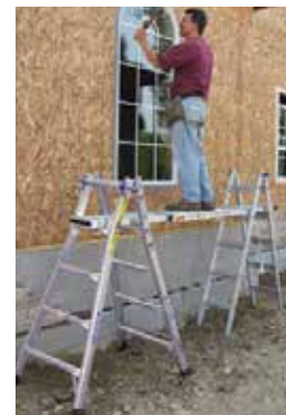
POSITION #4 Self-Supporting 2-Scaffold
